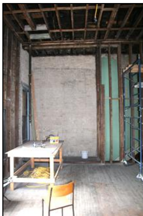
Kitchen will be here, washrooms were here.
