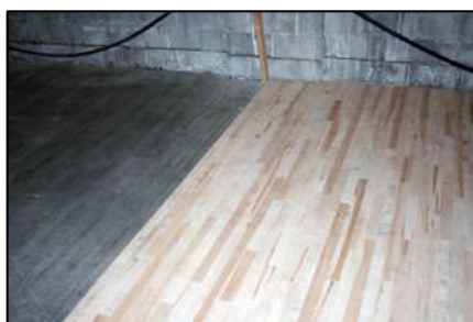
The new floor
