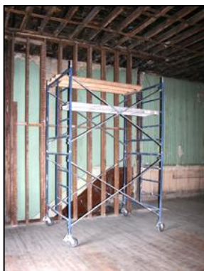
Dundas Street Stairway
