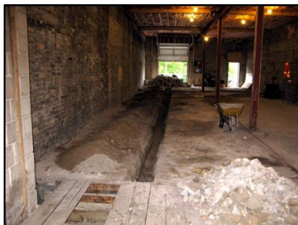
June 2009 – looking north to loading dock
