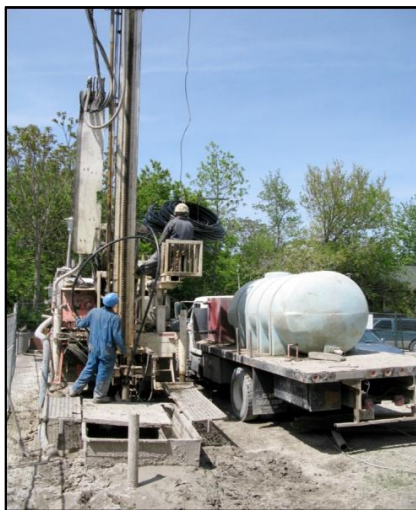
Drilling the geothermal field, May 2009
